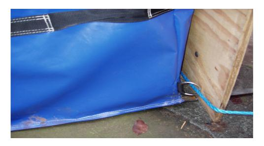
Securing the Barrier at the bottom with nylon rope
