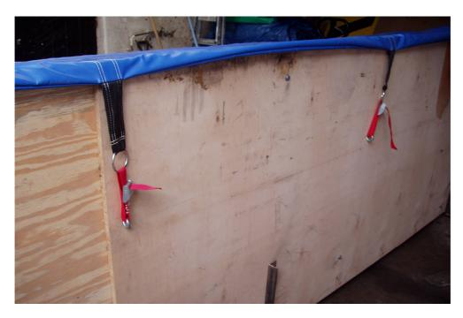
The 3.6 Metre unit is secured to the existing fence by 4 webbing straps. The back of the units are higher than the front to enable water to drain off the top of the unit.
